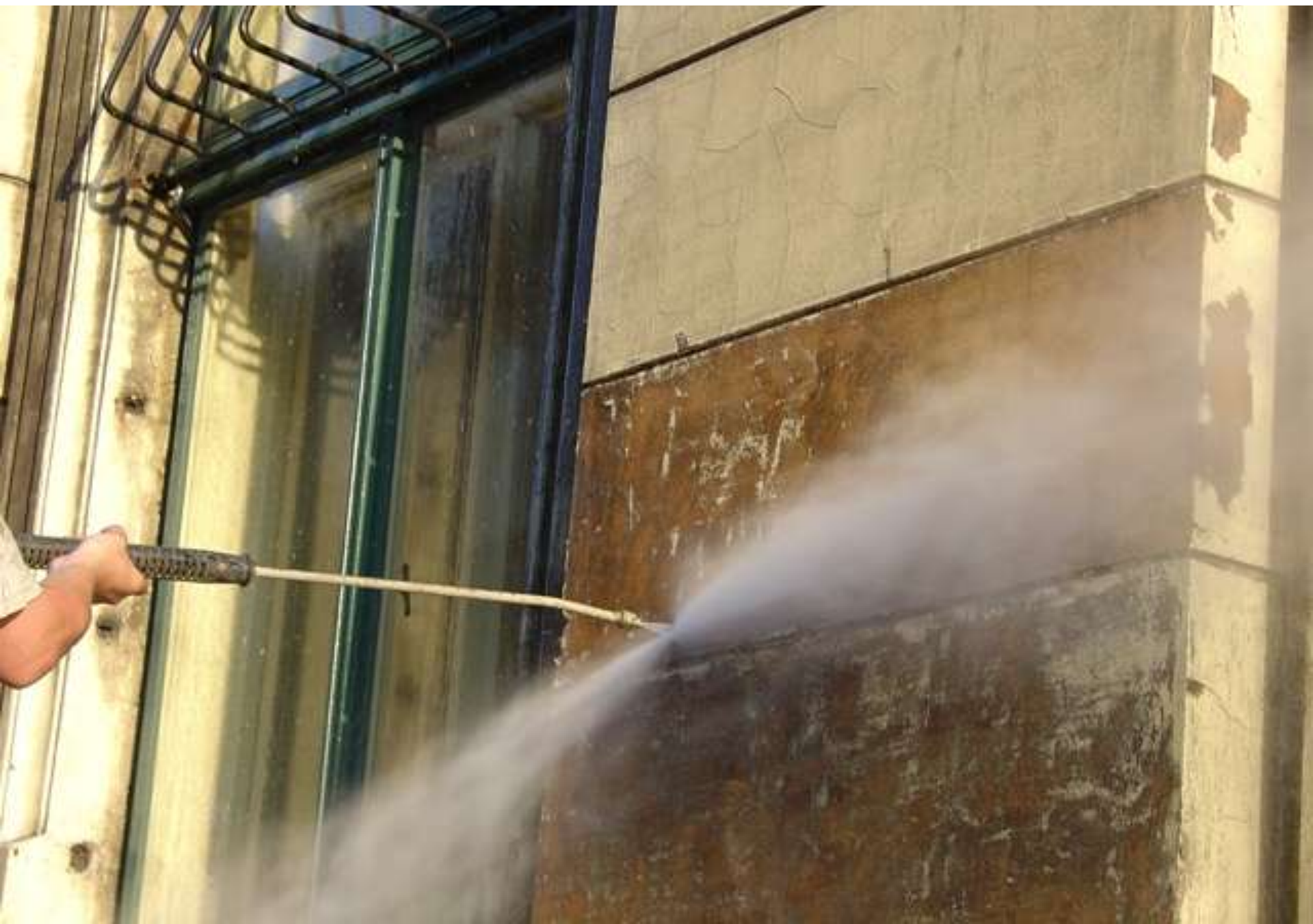
Cleaning with superheated water and sandblasting
