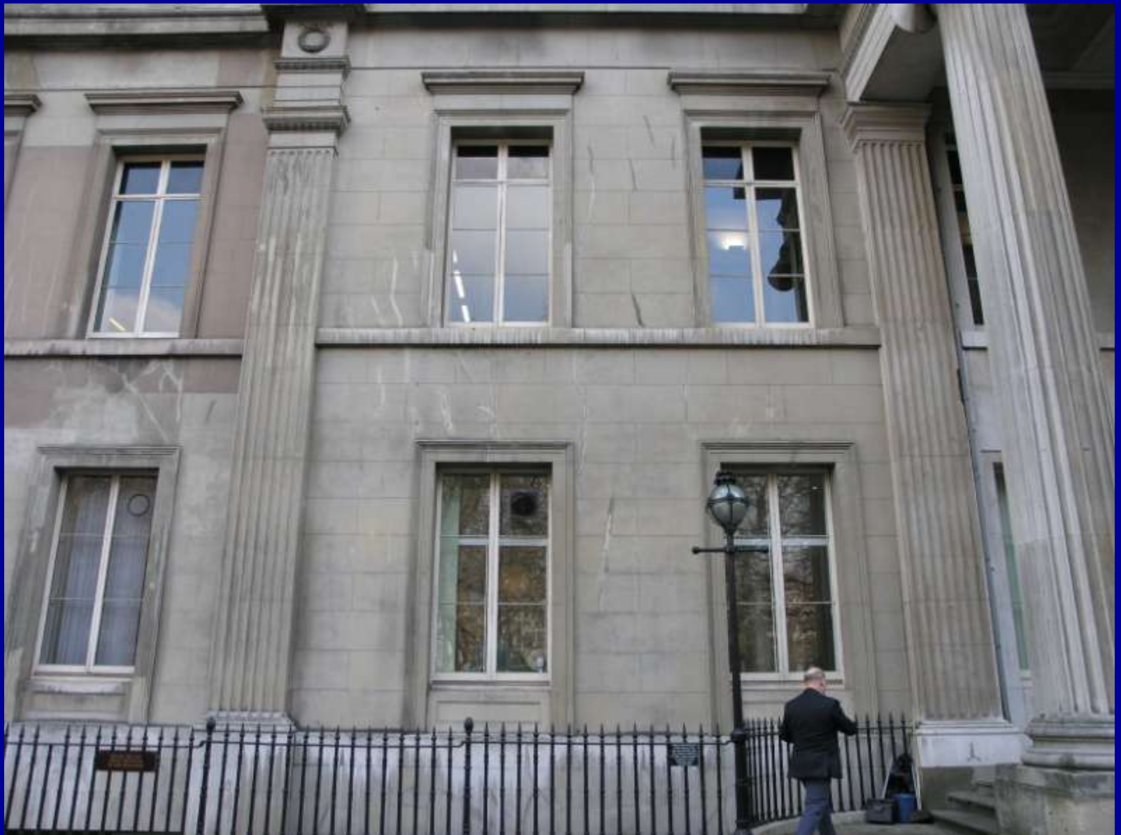
Royal College of Surgeons: William Ranger. Portico (predating the façade) in Natural Stone but the rest appears to be a mixture of stucco and casting.
