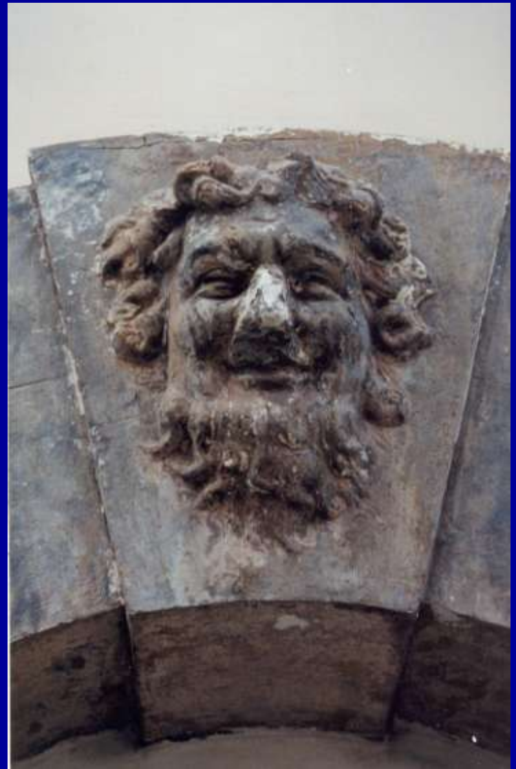
Cast Roman cement key stone in Woodbridge; probably by James Pulham, early C19th. ( an example of the use of Roman cement, not a Swann project).
