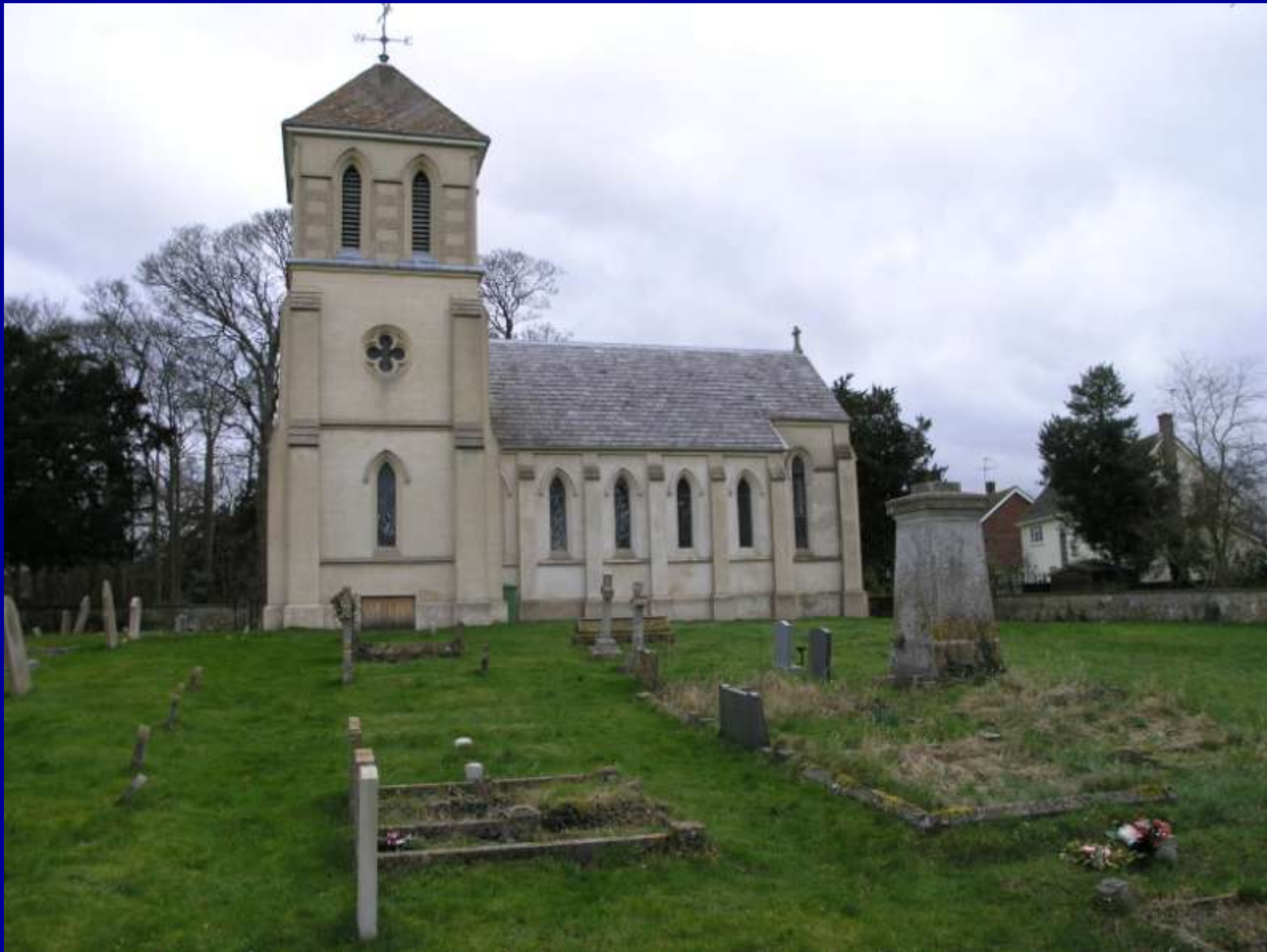
Westley Church: Suffolk, 1836, Lime mass concrete by William Ranger with cast ornament ( composition not known).
