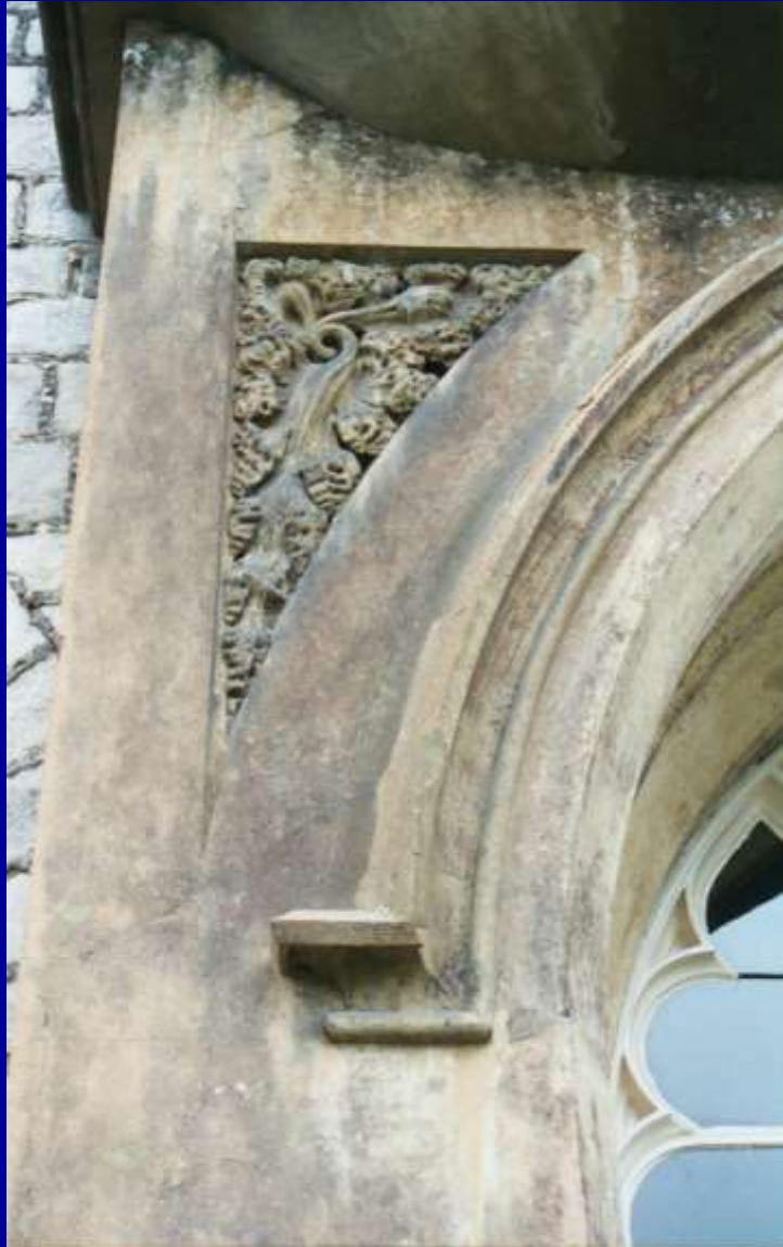
Wycombe Abbey, High Wycombe, Bucks. James Wyatt, 1804, in-situ run stucco and flat stucco window surrounds. Ornamental spandrels. Detail of RC work on East Façade.
