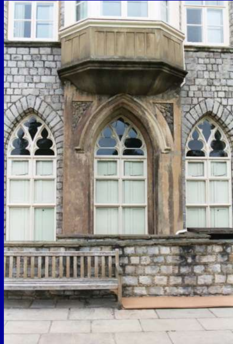
Wycombe Abbey, High Wycombe, Bucks. James Wyatt, 1804, in-situ run stucco and flat stucco window surrounds. Ornamental spandrels. Detail of RC work on East Façade.
