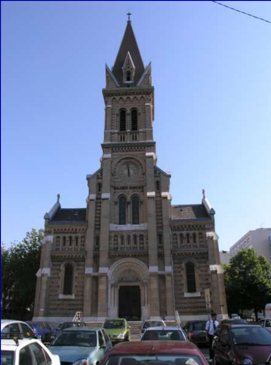
Eglise St Bruno, Grenoble, surfaced in cast natural cement artificial stone.
