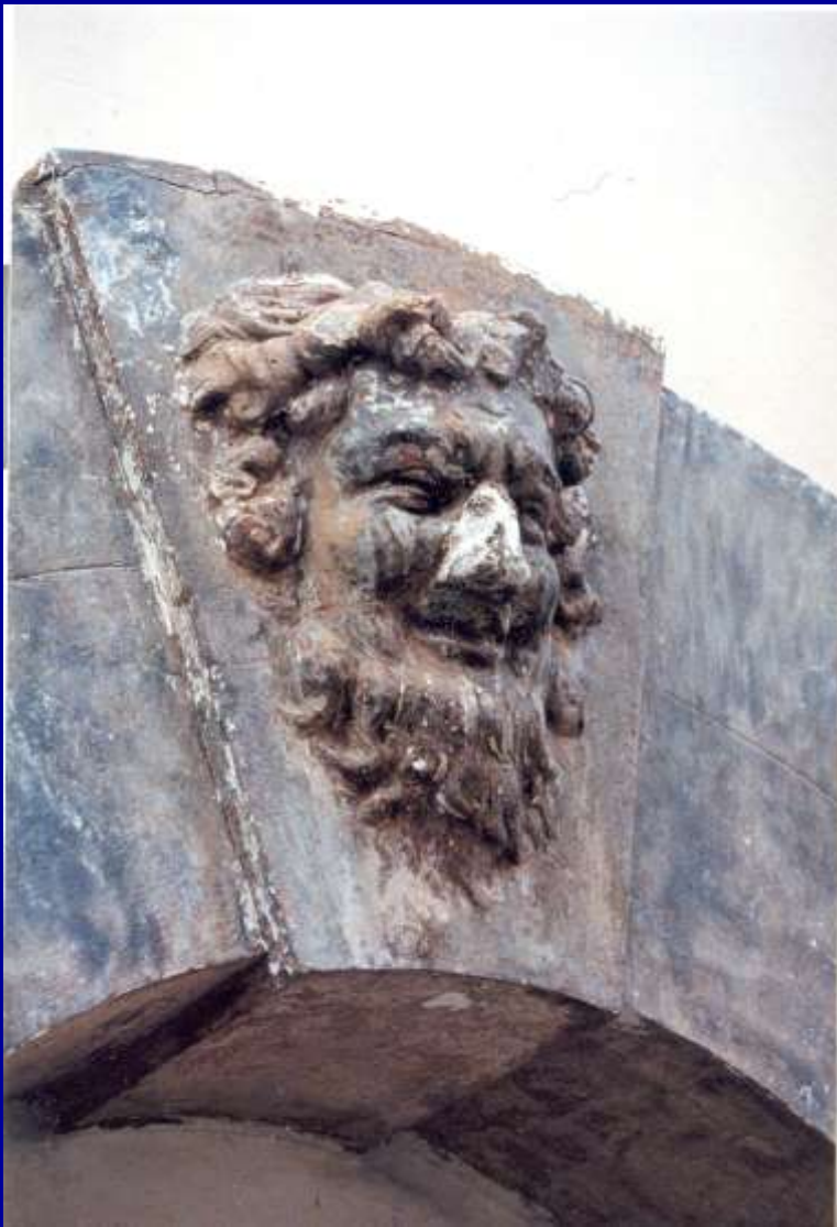
Cast Roman cement key stone in Woodbridge; probably by James Pulham, early C19th. ( an example of the use of Roman cement, not a Swann project).
