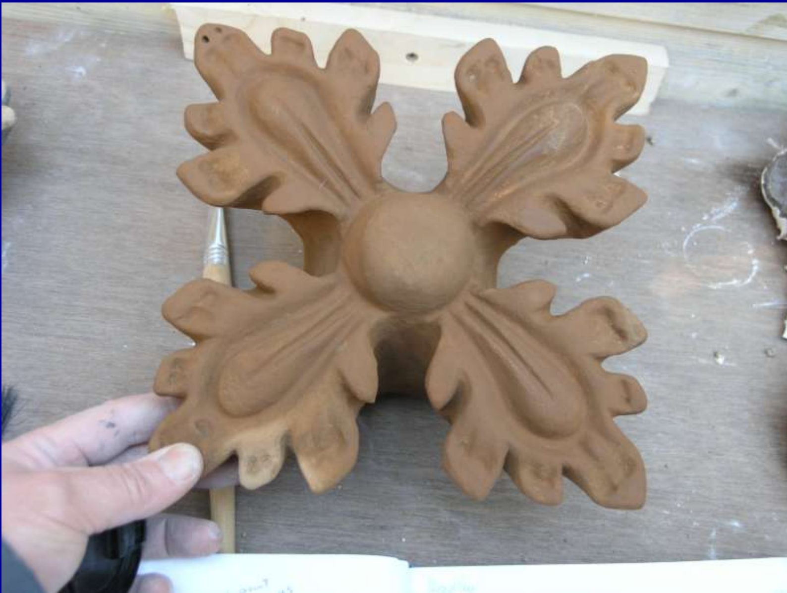
Hadlow rosette; conserved using prompt sand mortar for filling voids and prompt shelter coat for surface finish.
