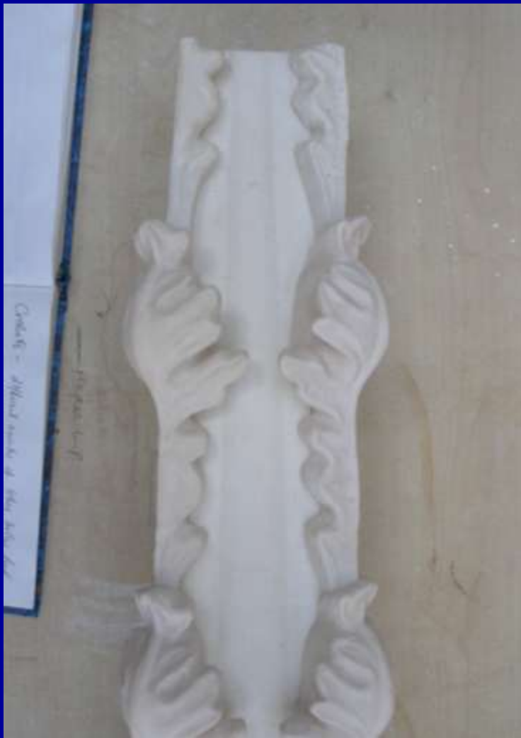
Hadlow Tower; small part of spirelet cast ( right) and complete replica for mould making.
