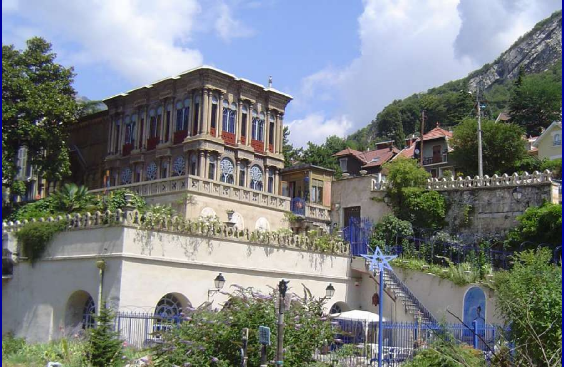
La Casamuères, St Martin le Vinoux, on the outskirts of Grenoble and not far from the site of Porte De France ( natural cement production from 1842). Casamuères was built from 1855 using extensive cast elements in natural cement.
