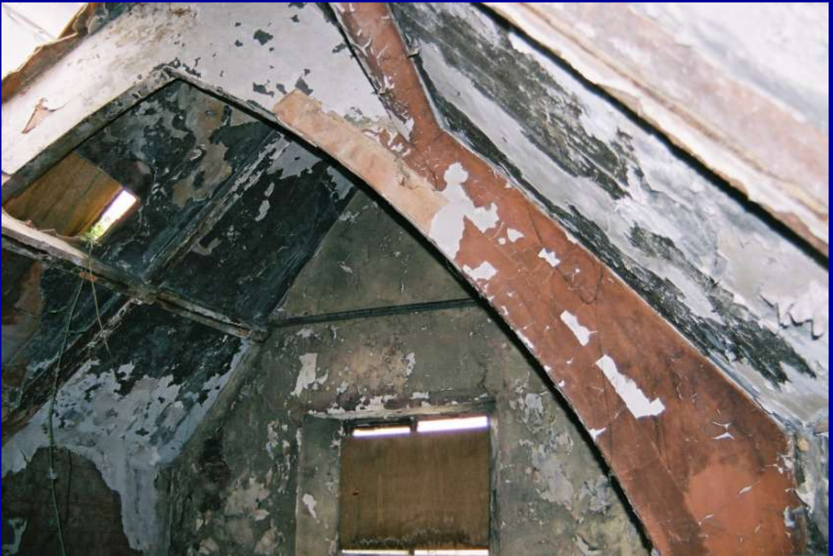
Detail from a room at back of Castle House with original cruck system still “intact” and tile creasing used for roof covering
