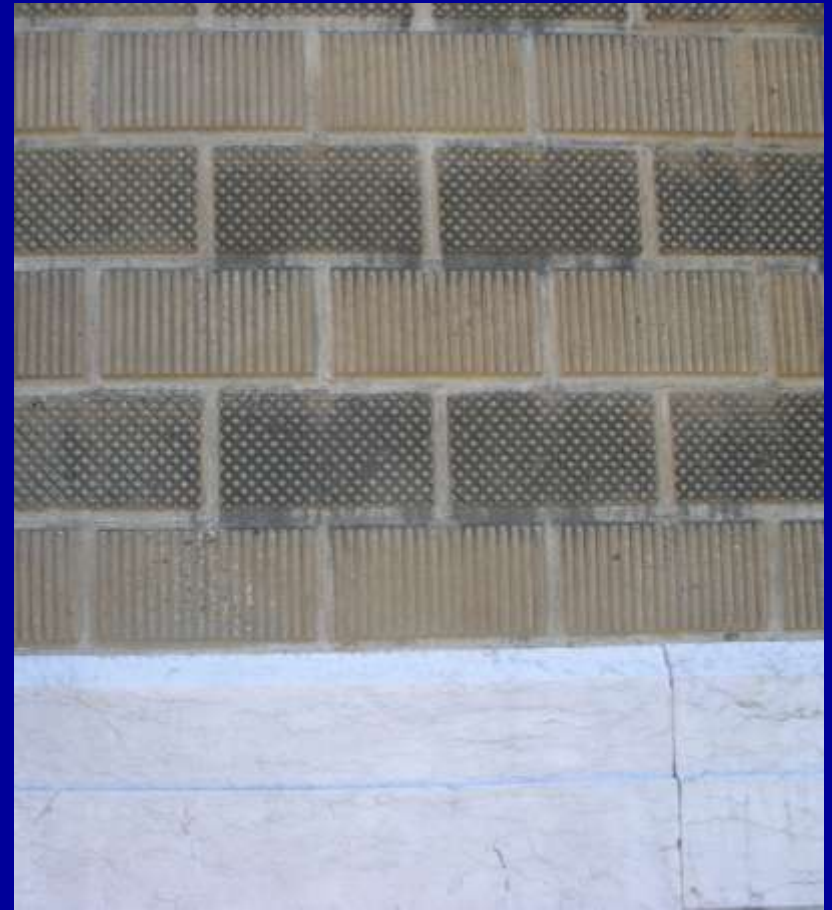
Eglise St Bruno, Grenoble, surfaced in cast natural cement artificial stone.
