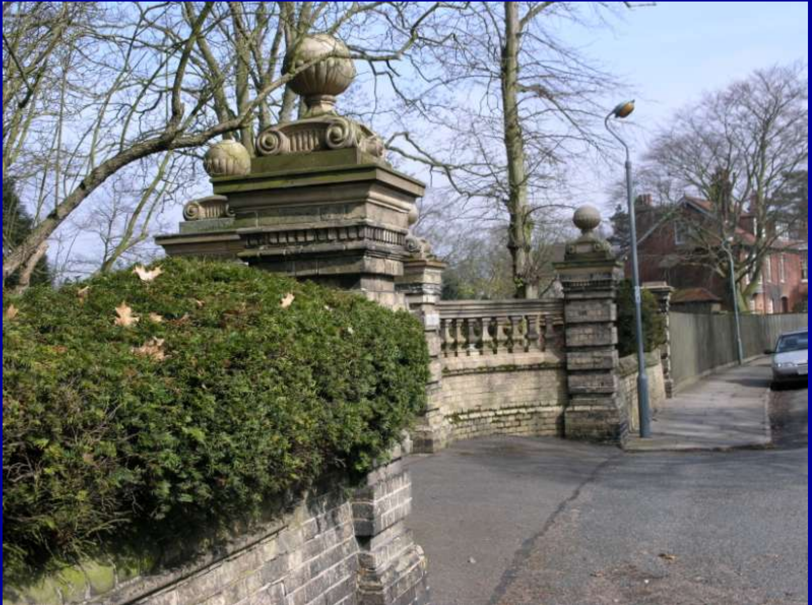
Constitution Hill, Ipswich; Suspected Ransomes Artificial stone; not all such castings were based on calcareous cements or lime. Ransomes work was based on dissolving flints and precipitating a silicate binder.
